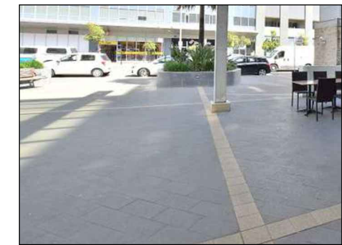
CODE: PV01 (PRIMARY PAVER) DESCRIPTION: PUBLIC DOMAIN PAVING TO MASCOT STATION TOWN CENTRE PRECINCT MASTERPLAN SIZE: 400x200x50/60mm FINISH: HONED EBONY WITH BLUESTONE AGGREGATE
