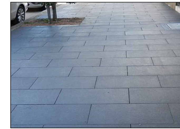
CODE: PV01 & PV02 DESCRIPTION: LARGE FORMAT TRAFFICABLE GRANITE PAVER SIZE: 600x400x60mm FINISH: EXFOLIATED
